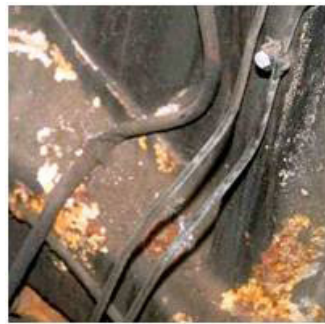
Figure 5. Engine compartment of 1976 Volvo showing uncorroded copper-nickel brake lines.
