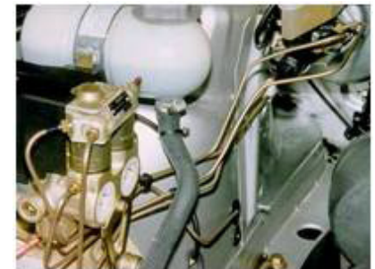
Figure 1. Copper-nickel brake lines running from master cylinder in 1990 Volvo.
